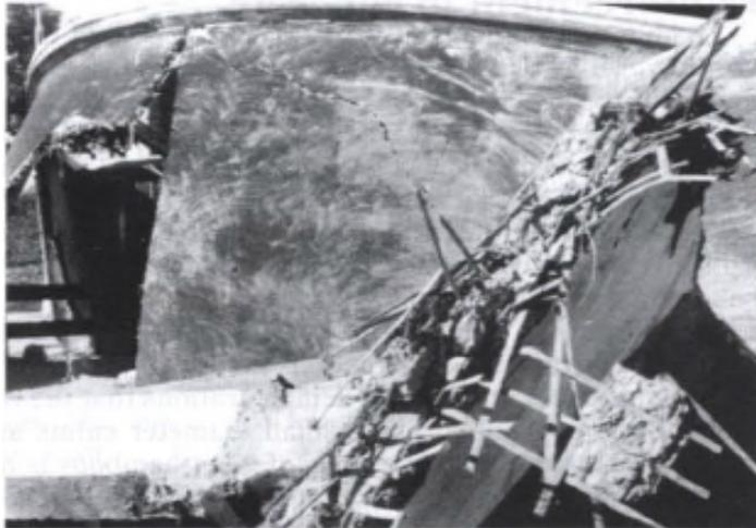
**C.** *There was a lack of adherence between the concrete and the bamboo reinforcement*
