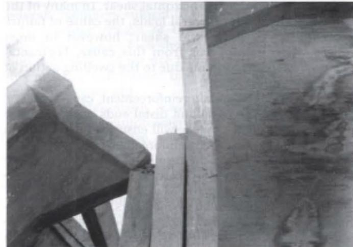
**D.** *The Bamboo reinforcement of the column broke.*
