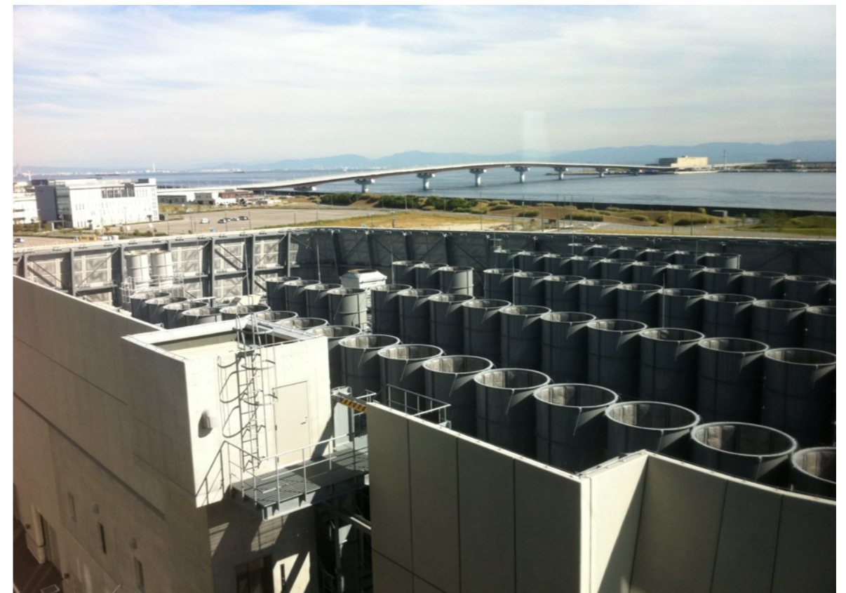
The K supercomputer in Kobe, Japan has an installed cooling capacity of almost 30 MW. October 4, 2011. Photo: Gerhard Schmitt
