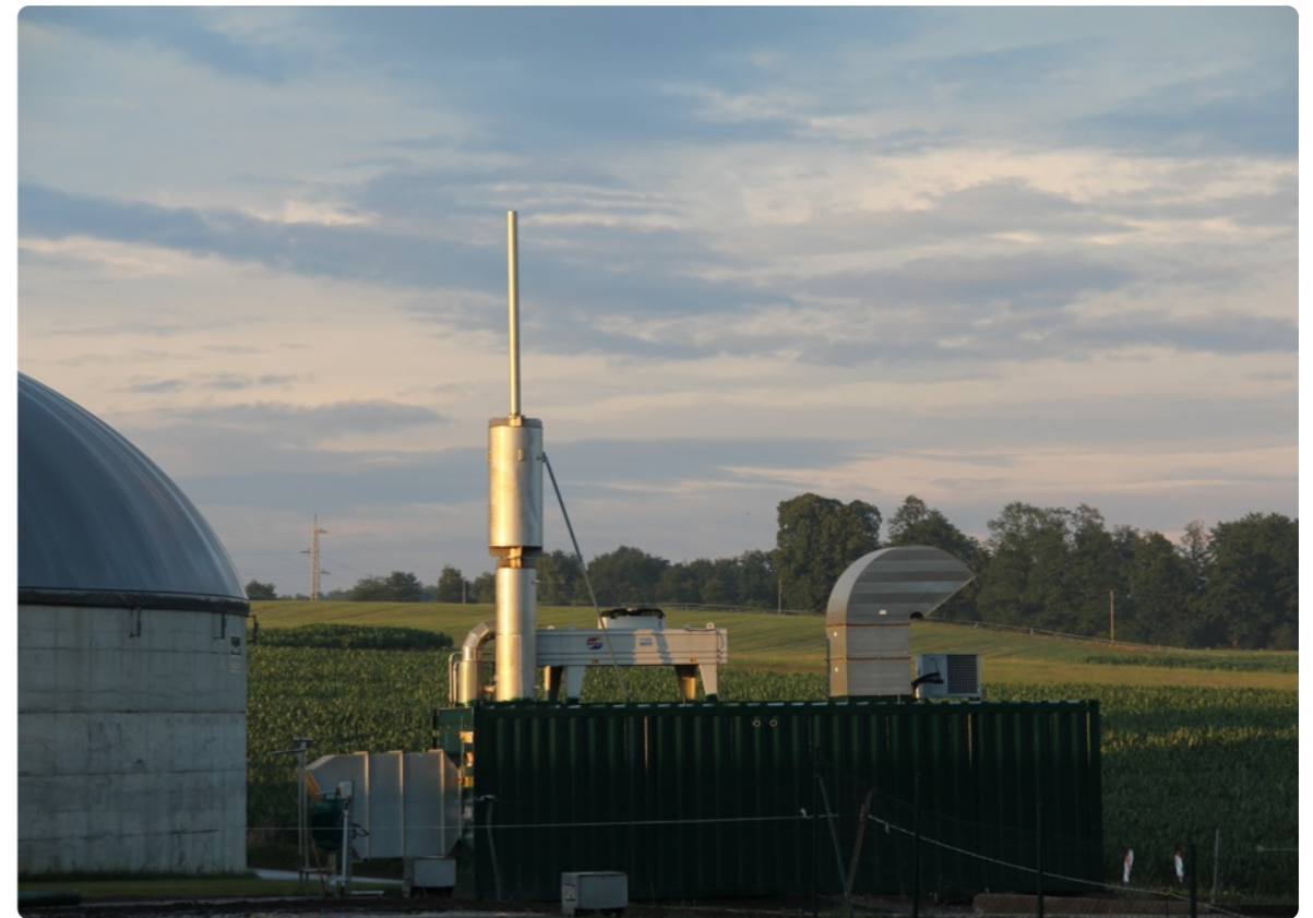
A 265 kW biogas plant supplying electricity for a part of a small town. Kastanienhof, Wadern, Germany, July 11, 2011. Photo: Gerhard Schmitt.
