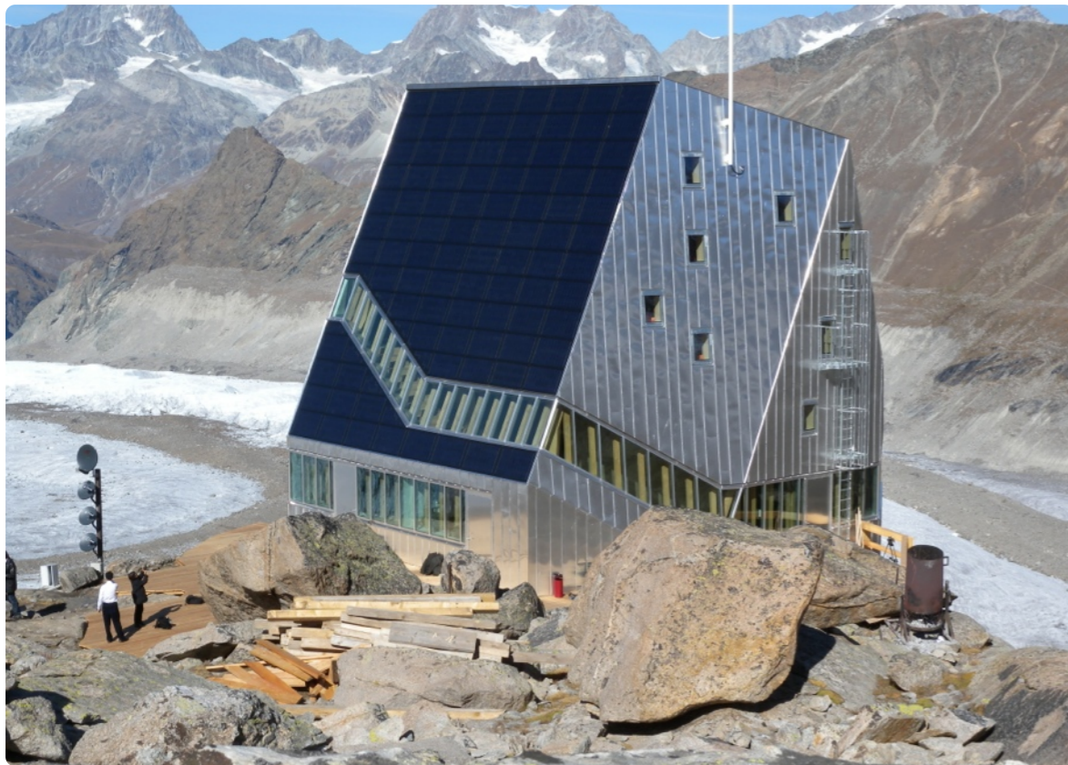
The Monte Rosa shelter produces all of its electricity with photovoltaic elements. October 3, 2009. Photo: Gerhard Schmitt.
