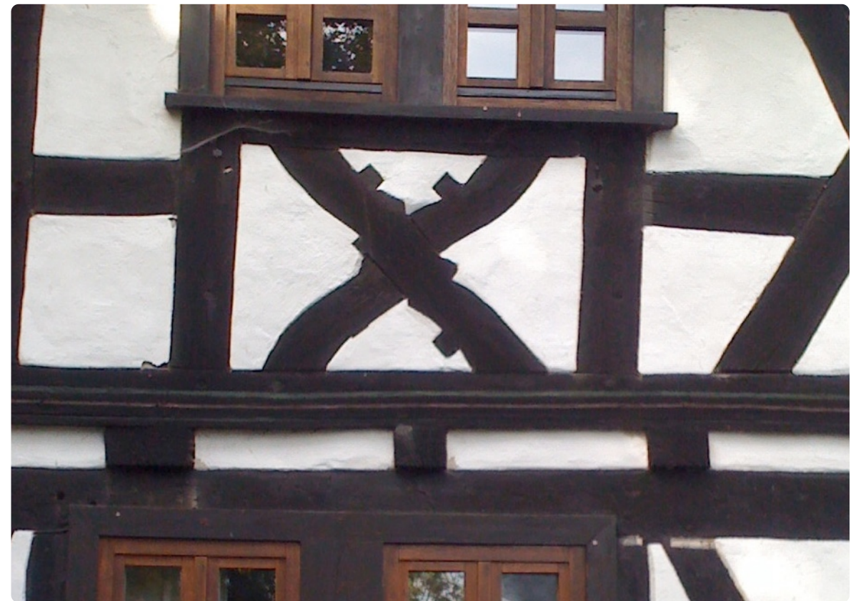
Oak wood, with adobe and straw infill. These local materials help sustain this schoolhouse in Schönberg since 1697. Photo: Gerhard Schmitt, October 10, 2008.
